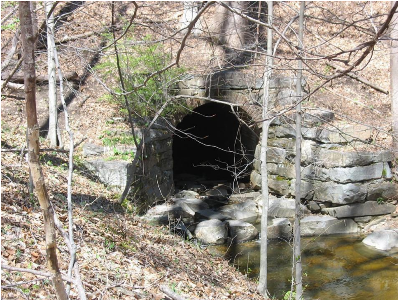
An Original O & A Railroad Culvert Photo by Michael DeLoose
